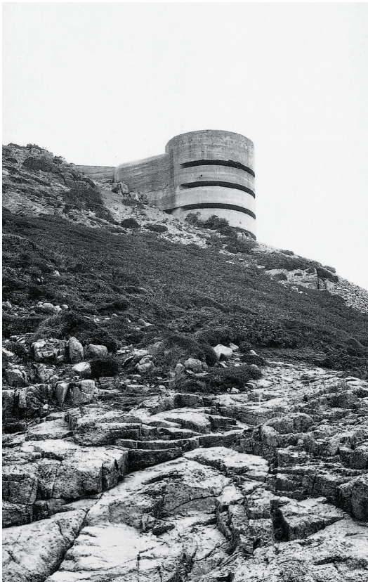
From top: Firing control tower, Landes, France, ca. 1958–65. Observation post, France, ca. 1958–65. Photos: Paul Virilio.
